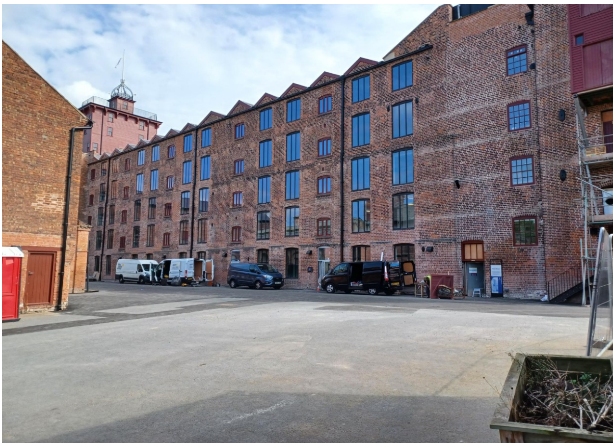
- West View of shop door entrance –
