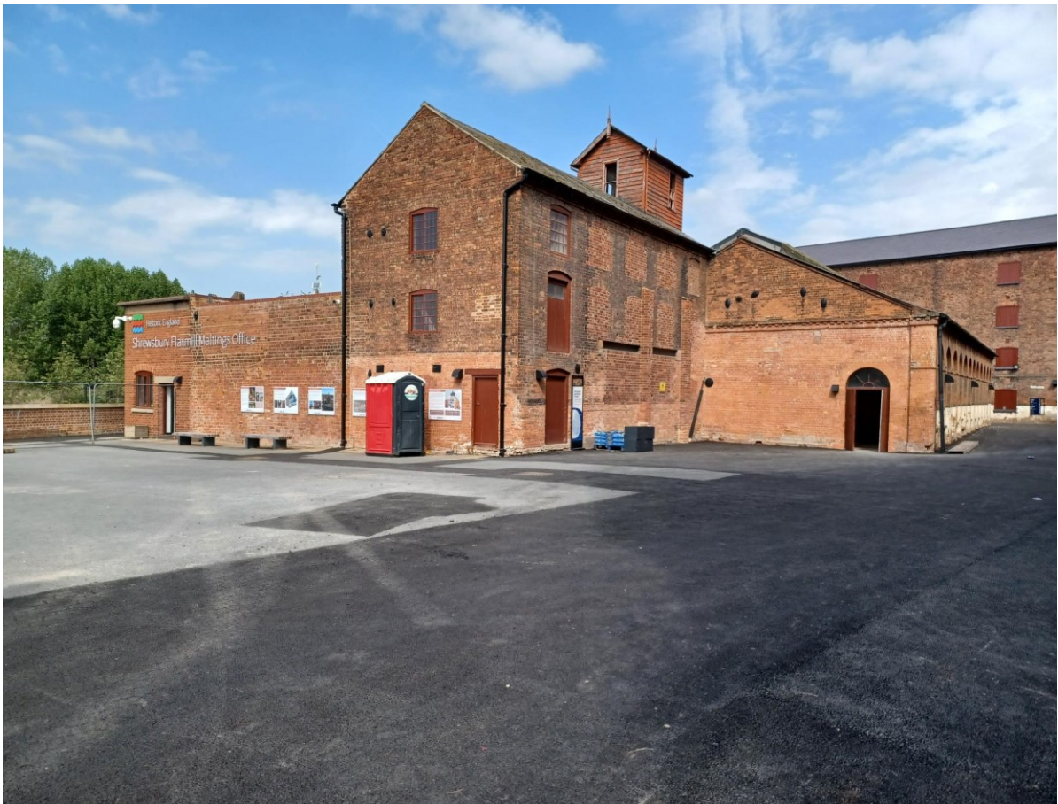
- Dye House to the right, with office to the left -
